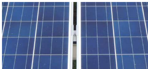
Figure 7: 50mm (2 inch) mid-clamps
